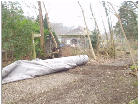
Photo 2- laying of Fibretext material onto existing subgrade
