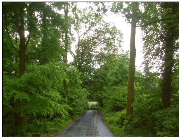
Photo 5- completed road using porous tarmac surfacing
