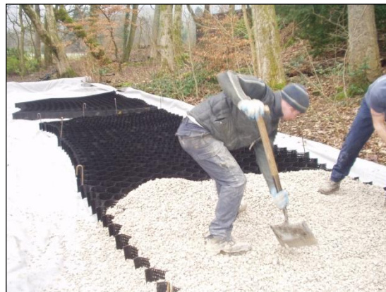
Photo 3- expanding and filling the Cellweb system
